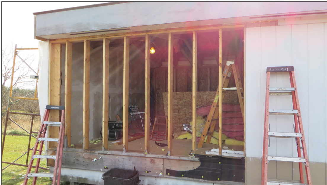
Figure 2. Northeast corner of test structure undergoing partial reconstruction.
