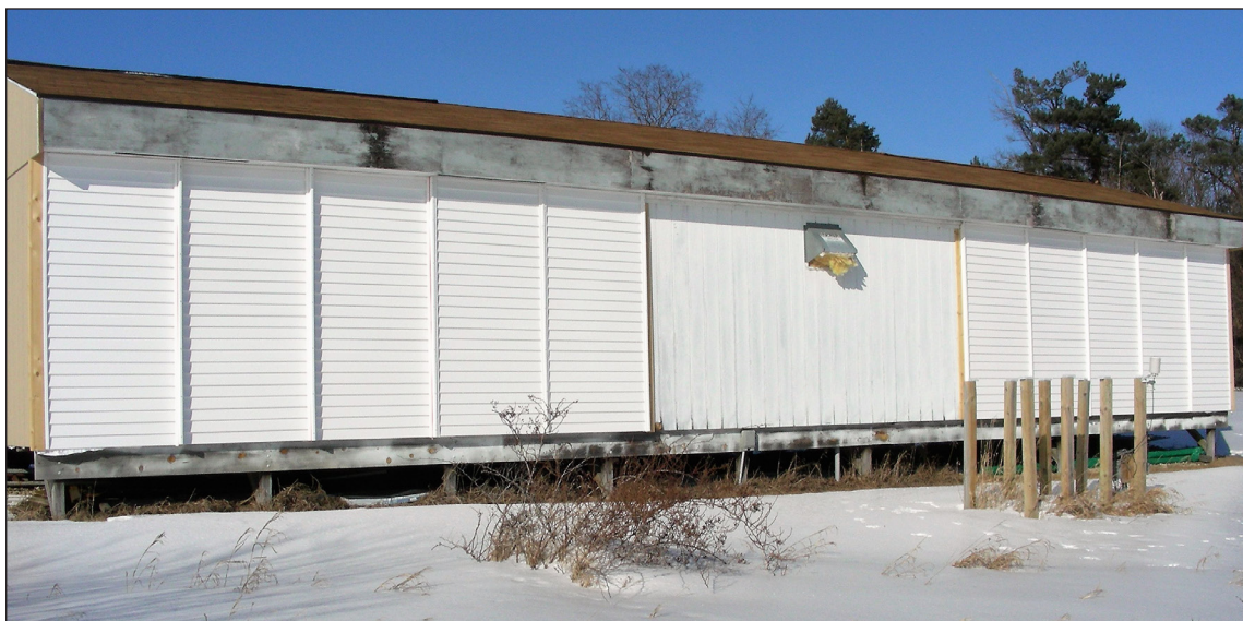
Figure 5. Completed south side of the test structure.
