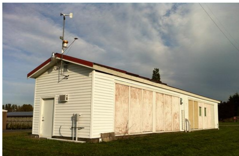
Figure 2. NET facility viewed from the southwest
